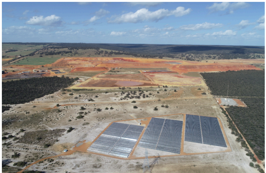
The 3MW Solar Farm and the Mine in the background.
