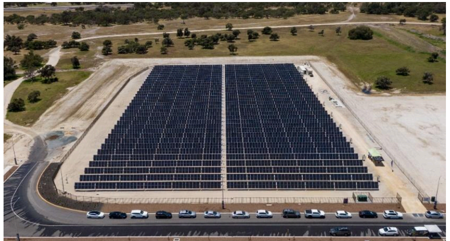
Photo: Solar farm shortly after installation of panels Dec-2020
