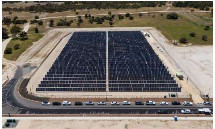
Photo: Solar farm shortly after installation of panels Dec-2020
