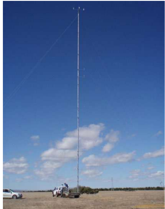
Figure 4 Typical 60m Monitoring Mast
