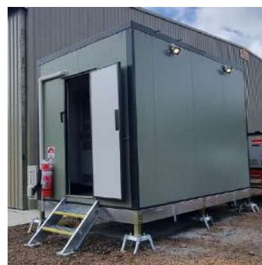
Custom Built Plant Room for the BESS
